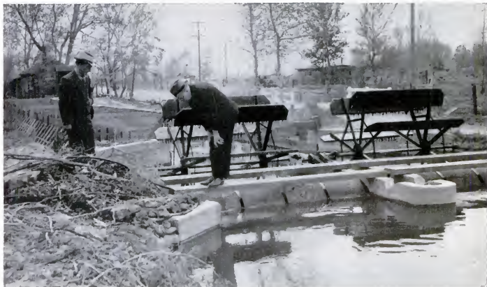
Young salmon are detoured away from irrigation canals by these screens, which revolve to avoid being clogged
